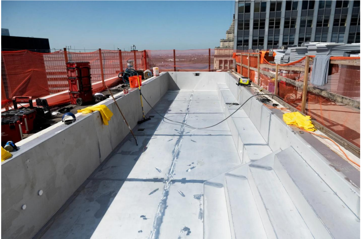
The rooftop pool under construction. Photographer: Stephanie Keith/Bloomberg
